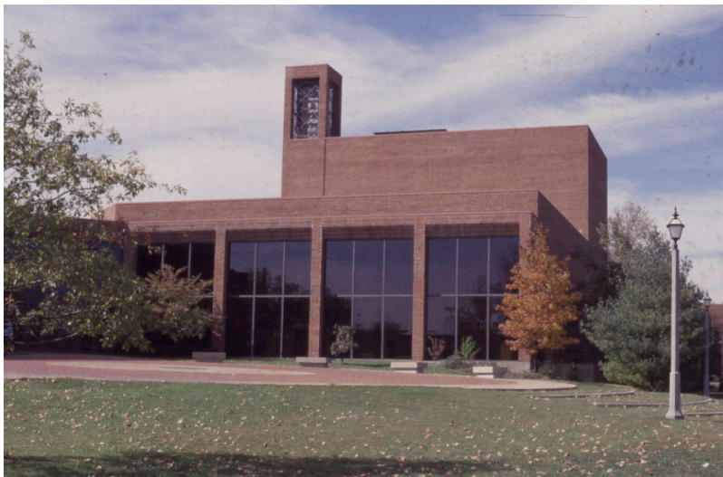
Figure 3.2: Performing Arts Center 35
